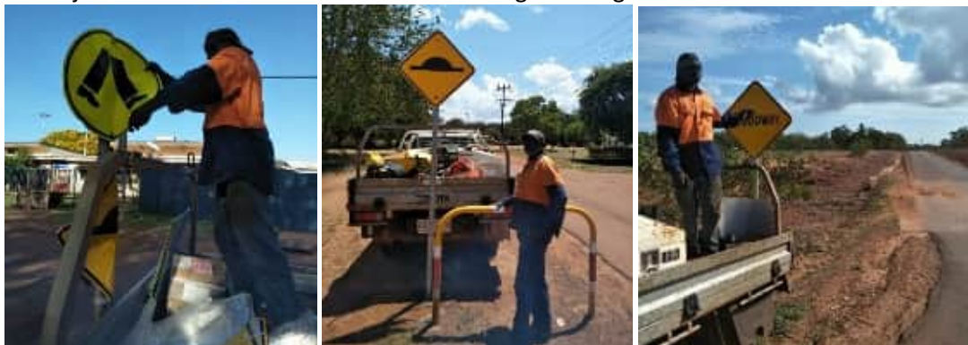
Installation of road signs throughout the Maningrida community.
